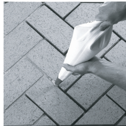
Figure 16 - Grouting Brick
